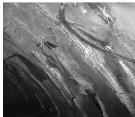
Figure 1: View of the location, in which a massive penetration of moisture occurred: new solid-carbonate formations are visible on the surface of the lining
