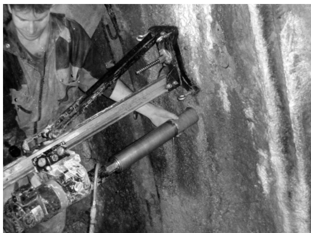
Figure 2: Collection of core bores from the lining. Significant carbonate efflorescence is visible on the surface of the wall.
