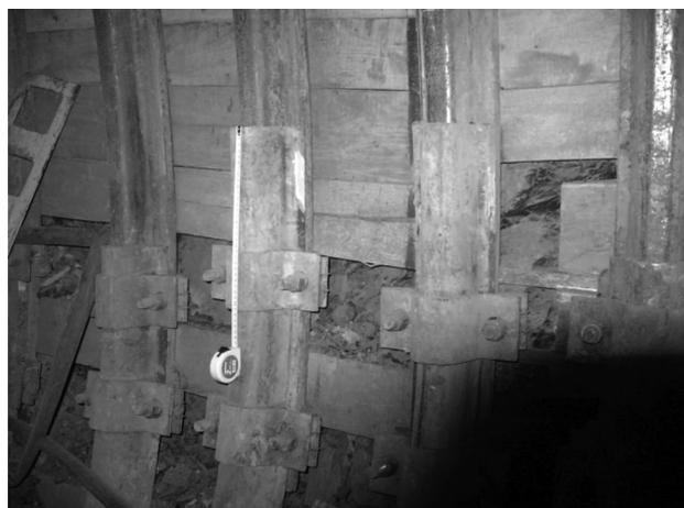
Figure 7: Damages on K24 support after a rock burst
