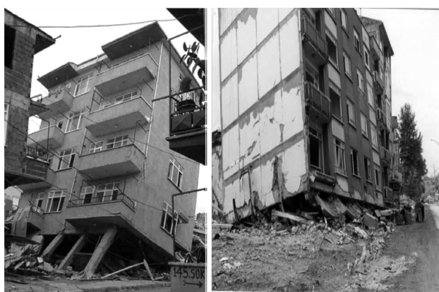
Figure 1: Soft-storey damage 1
